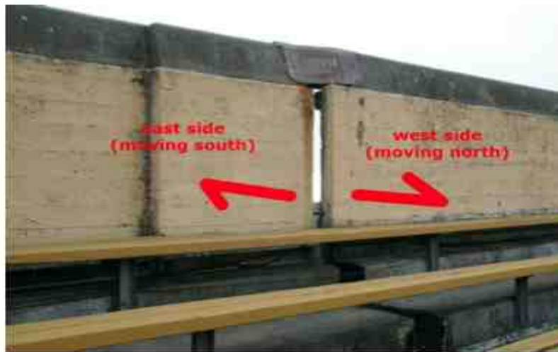
Offset of rim wall of California Memorial Stadium from Hayward fault, section KK, Row 64 offset of 7" between seats 22 and 23 from Stoffer 2008.
