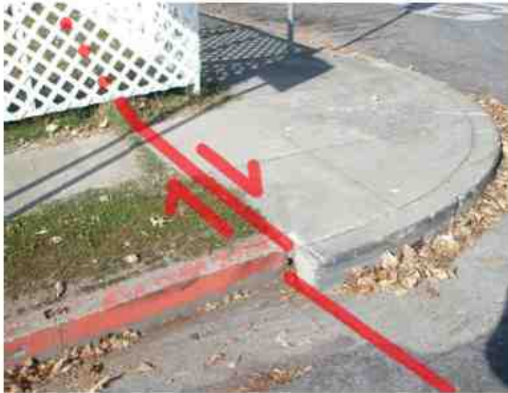
Offset curb at Prospect St and Rose St downtown Hayward showing right-lateral displacement from Stoffer 2008.
